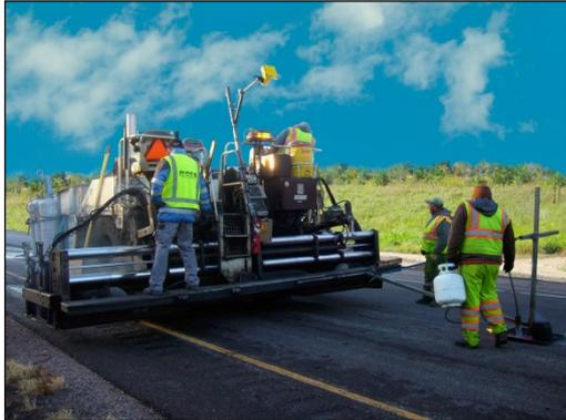
*The temperature scanner measures the temperature of the asphalt over a width of up to 13 meters depending on the measurement angle and mounting height*
